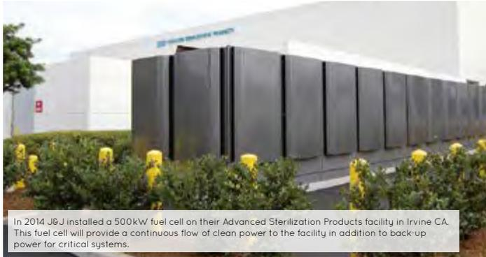
In 2014 J&J installed a 500kW fuel cell on their Advanced Sterilization Products facility in Irvine CA. This fuel cell will provide a continuous flow of clean power to the facility in addition to back-up power for critical systems.
