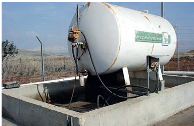
Effective containment of a tank
